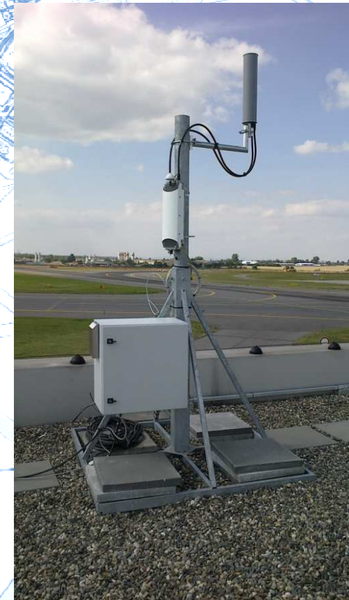
Figure: Installed BS with antenna
